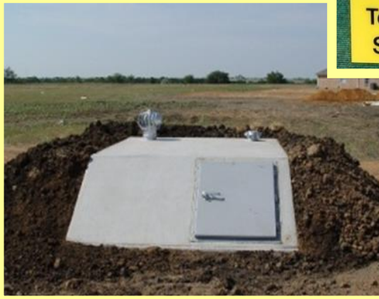
Concrete Underground Storm Shelter
